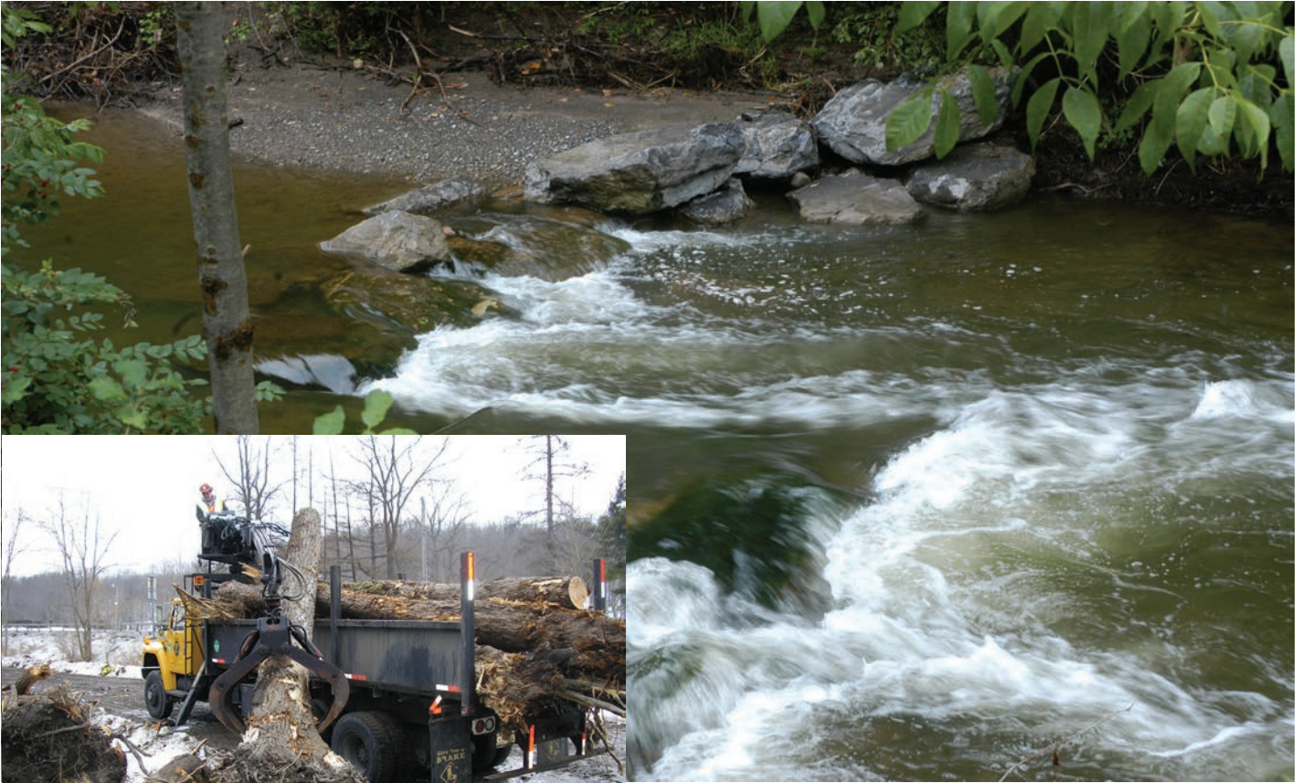
Stream improvement involved placing boulders (above) and root wads (left) to combat stream bank erosion (bottom) and improve trout habitat. NYSDOT partnered with DEC and provided many of the trees used in the project.
